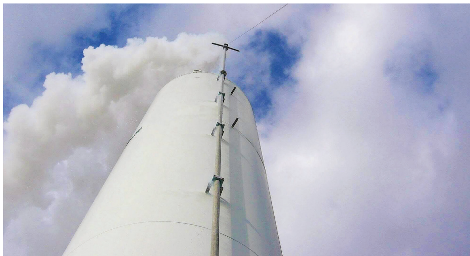
Typical bulk storage tank venting GH 2 to relieve pressure. Hydrogen venting losses can exceed 20%, with actual 'real-world' losses at or near 40%. Credit: GenH2
